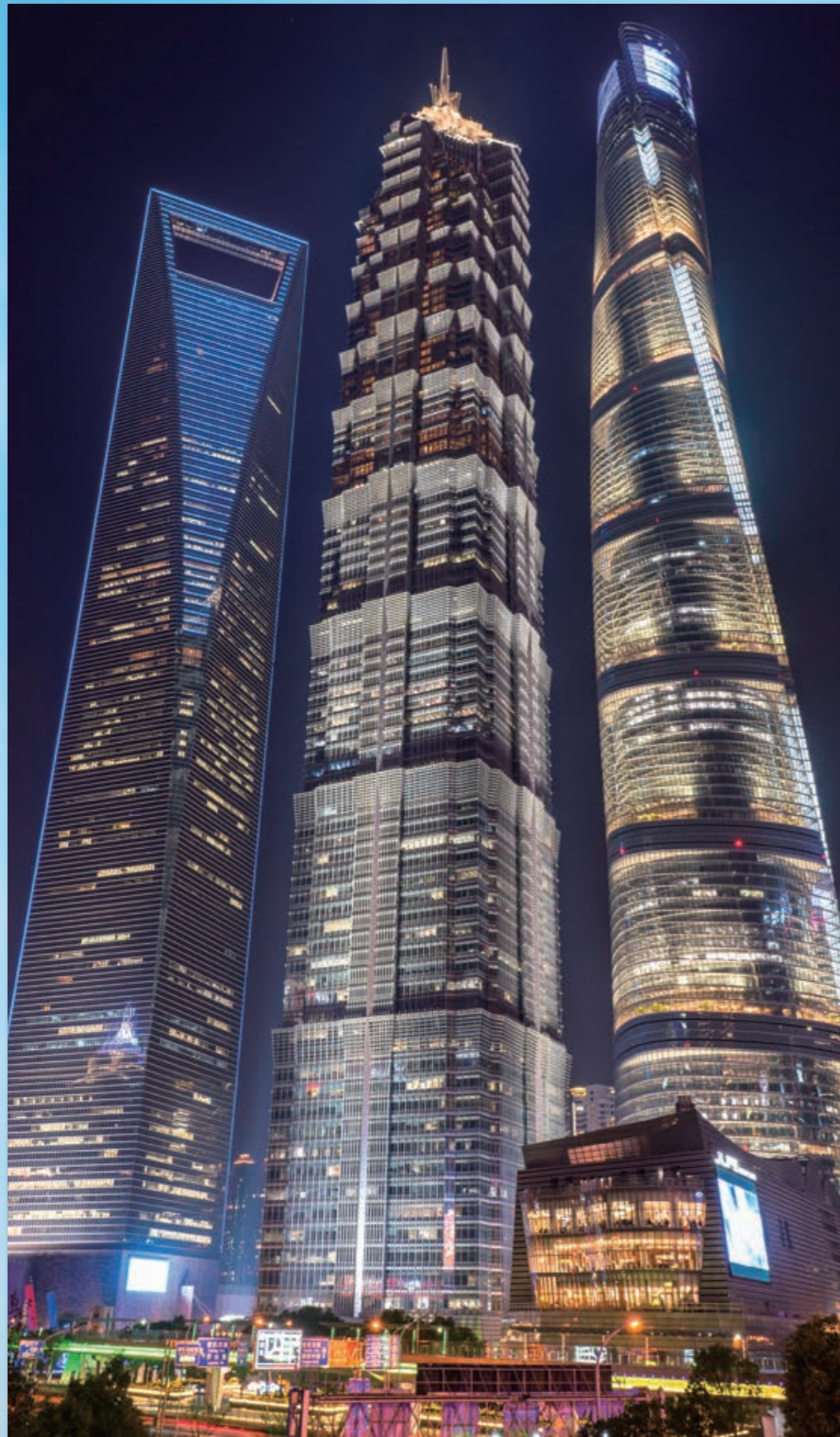
Shanghai World Financial Center, Jin Mao Tower, Shanghai Tower (China)
