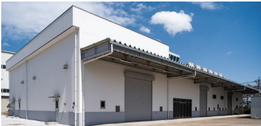
<Exterior of the Air Conditioner Comprehensive Testing Facility at the Kanagawa Factory>
