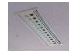
UV-C lamp-equipped fan coil unit (patented)
