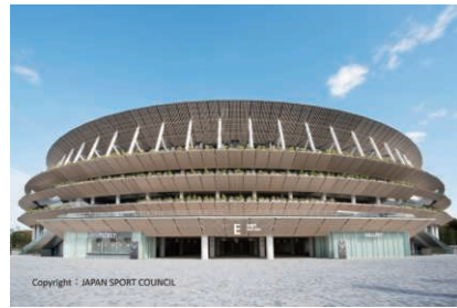
Japan National Stadium
