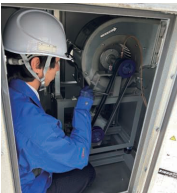
V-belt tension measurement
