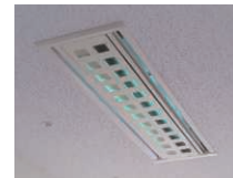
UV-C lamp-equipped fan coil unit (patented)
